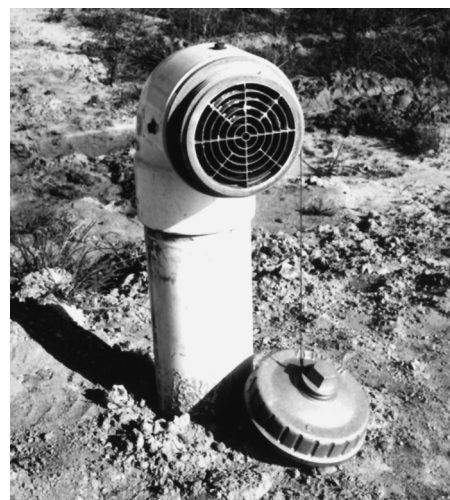
FIGURE B.8.1 Dry hydrant.
