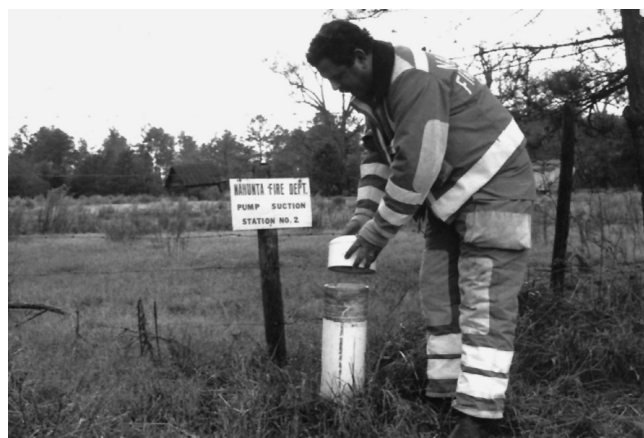
FIGURE B.8.3(a) A dry hydrant innovation has eliminated the top 90-degree or 45-degree elbow on each hydrant. (Photo by Nahunta Volunteer Fire Department, NC)
