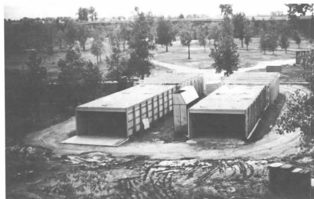
Figure 3(a) Overall view of 20-ft by 100-ft fire test building from exhaust end.
