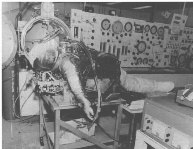
Figure 3-2.6.7 A fire occurred in which this space suit was destroyed. No one was in the suit at the time of the fire. (Photo courtesy of NASA/Johnson Space Center)
